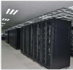
Computer room monitoring
