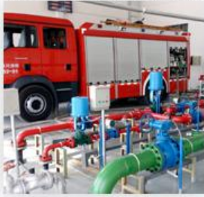
Fire Control System
